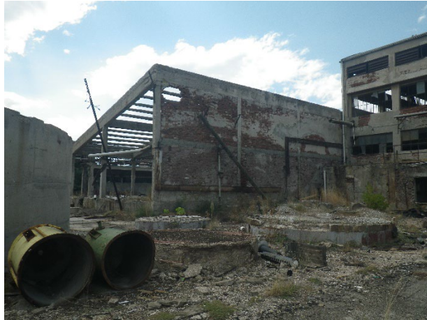
Figure 1 - Former mercury cell facility in North Macedonia
