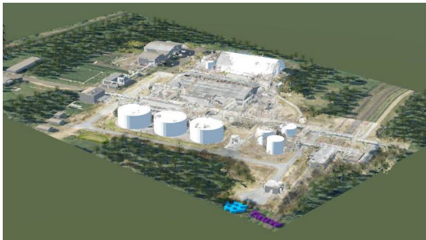
Figure 5 - 3D scan of Chlor-alkali site in Europe
